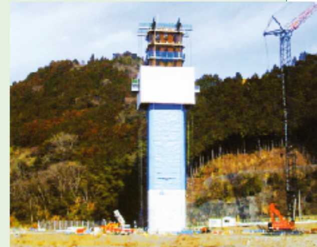
HSF (Hybrid Slip Form) method for High Pier
