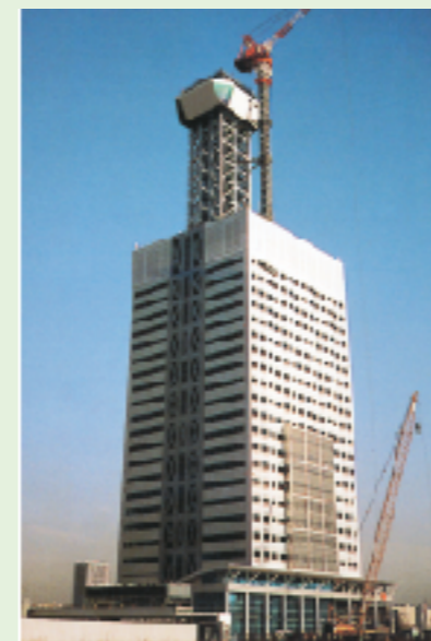
Climbing scaffolding method for M.M. DoCoMo Building
