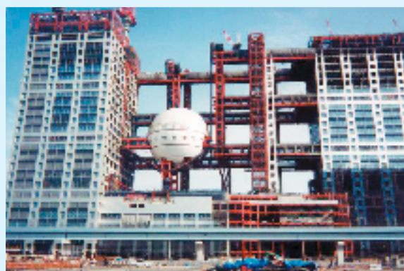
Fuji-Sankei Building (lifting weight: 1,200 tons)
