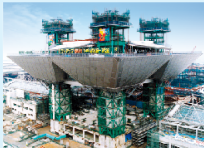
Conference building of Tokyo Big Sight (lifting weight: 6,500 tons)
