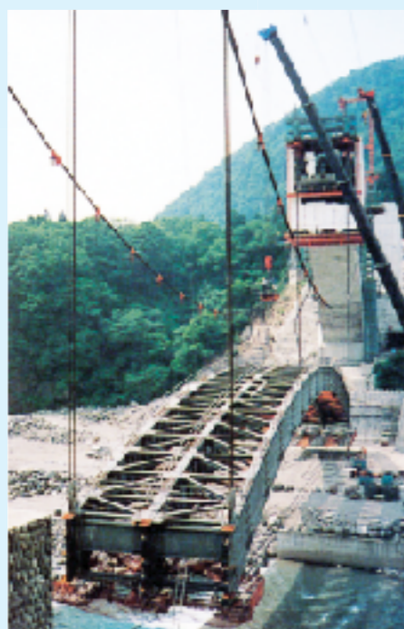
Melan arch structure of Gokuraku Bridge (lifting weight: 600 tons)
