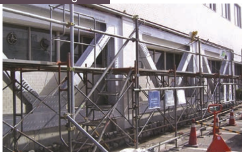
Nippon Kokan Hospital Outpatient Building seismic retrofitting project
