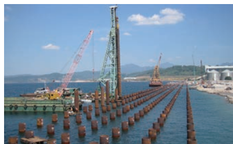
Pile driving for Subic Container Terminal (Philippines)
