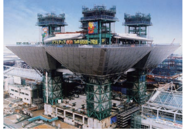
Construction of heavy facility by Jack-Up construction method
